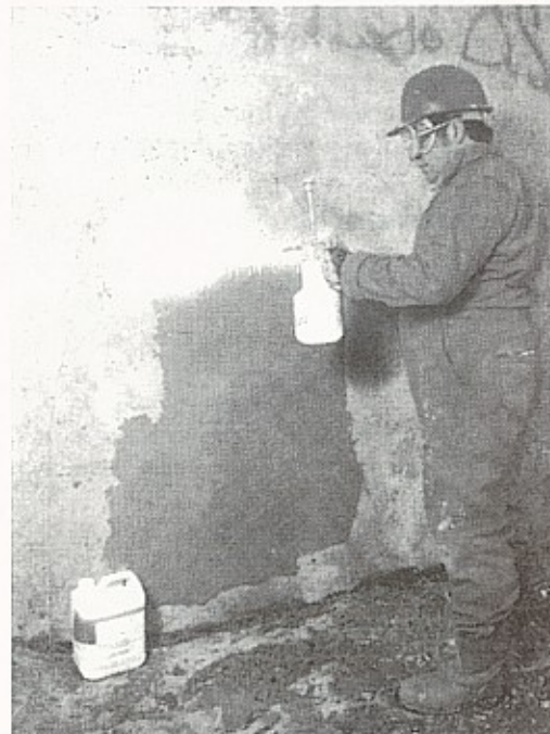
NITOBOND AR being applied to the area repair.
